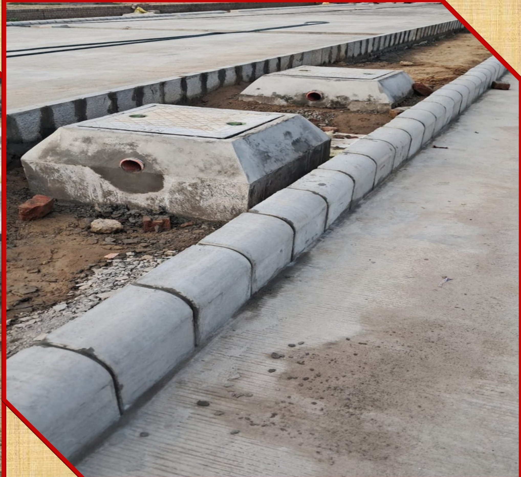
Kerb Stone , Saucer drain Fixing along side CC Road
