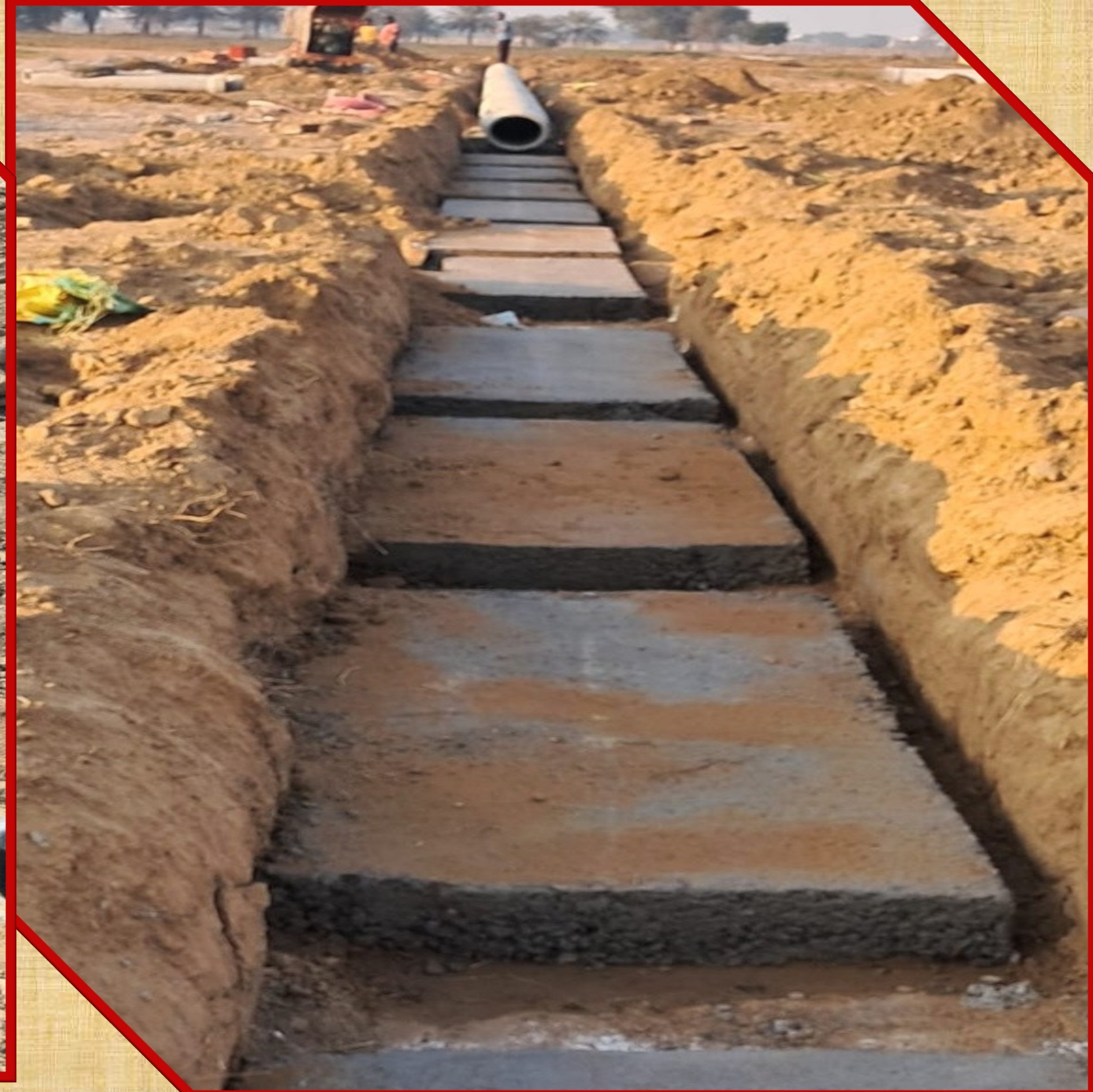
Sewerage Line Digging
