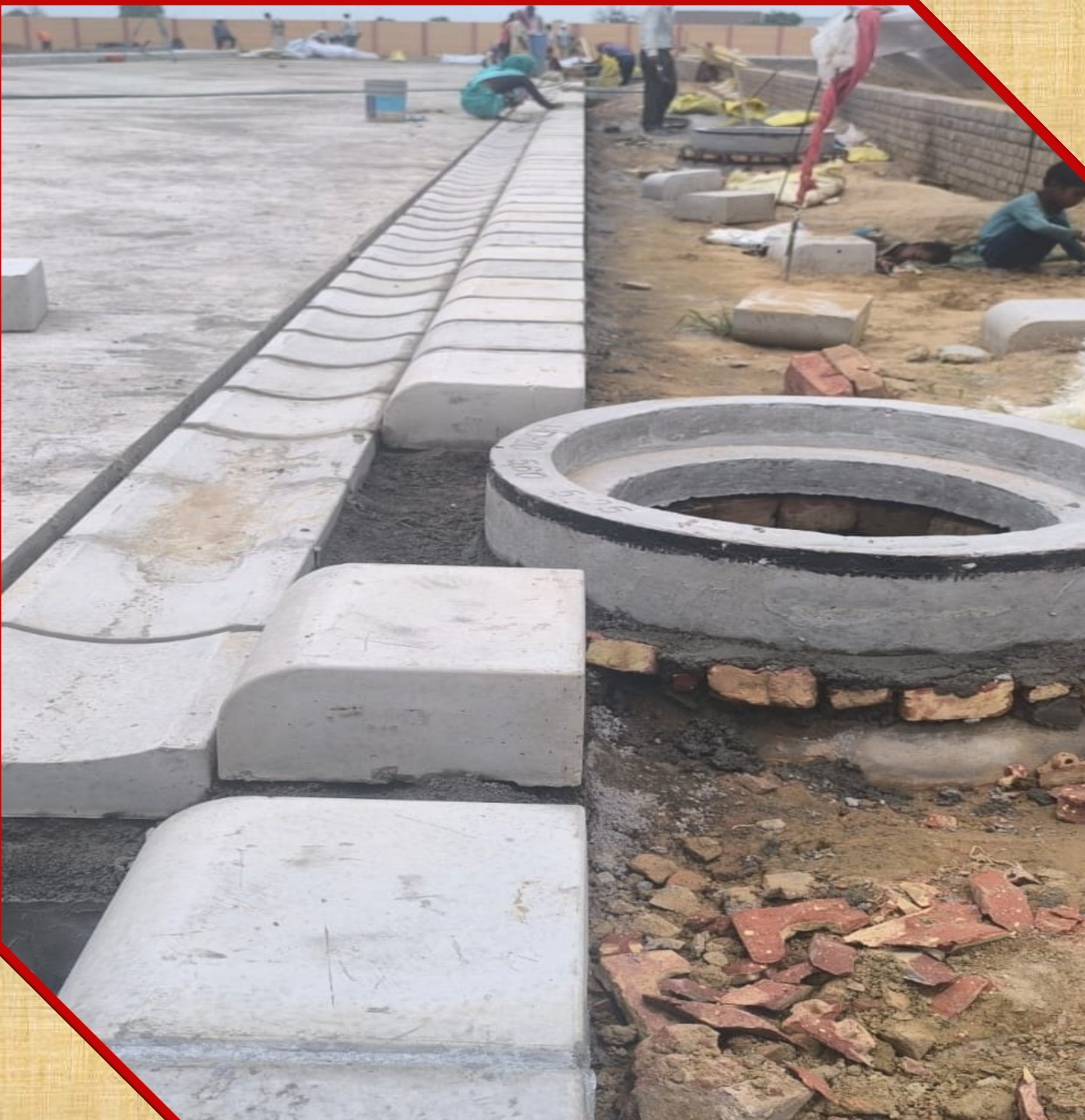
Kerb Stone , Saucer drain Fixing along side CC Road
